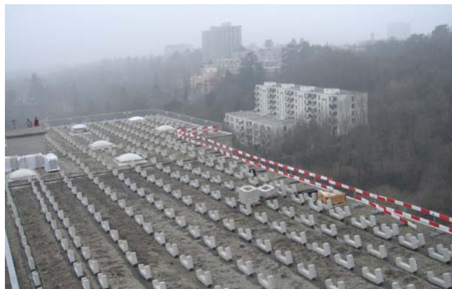
Construction of structure
