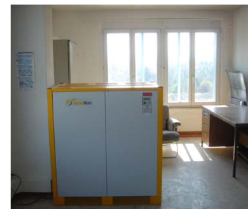
Solarmax 100 inverter
